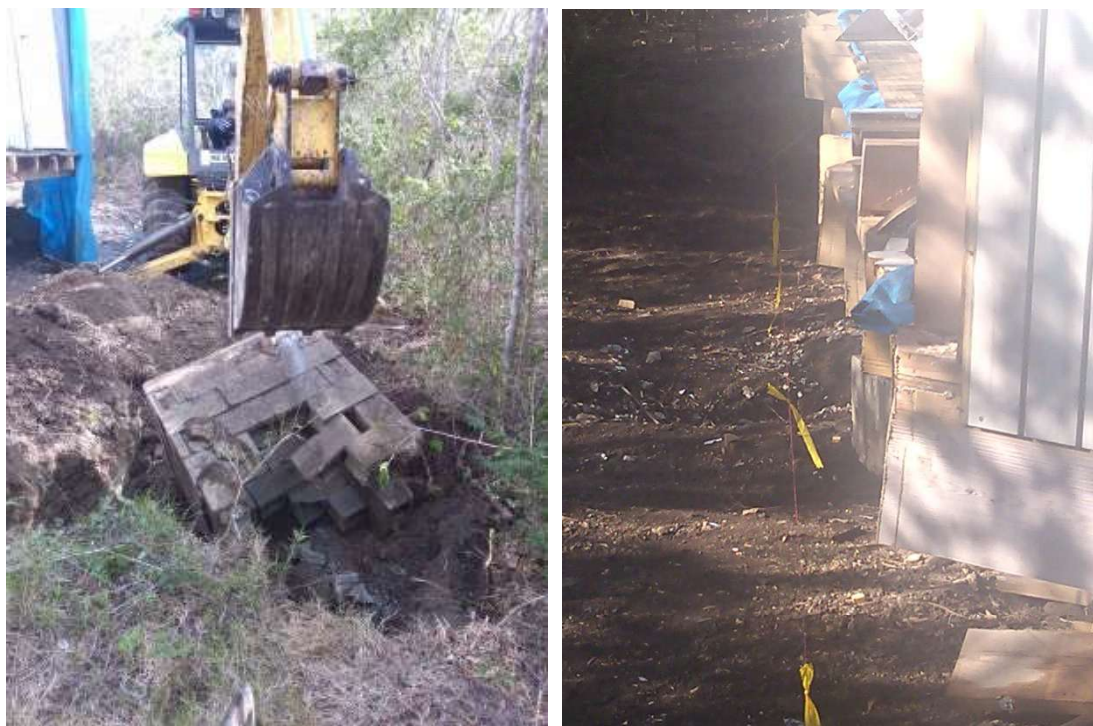
Figures 7B: Existing water tank and septic removed. The corner of the existing building was cut off at the property, prior to my acquisition of 19 Susannaberg (photos taken April 2013).
