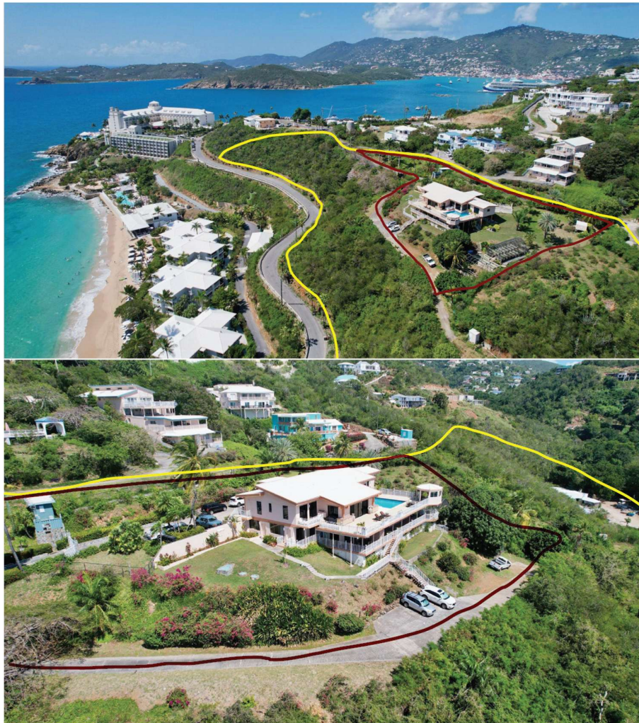
Site photo- subject properties outlined in red. Adjacent owned properties outlined in yellow
