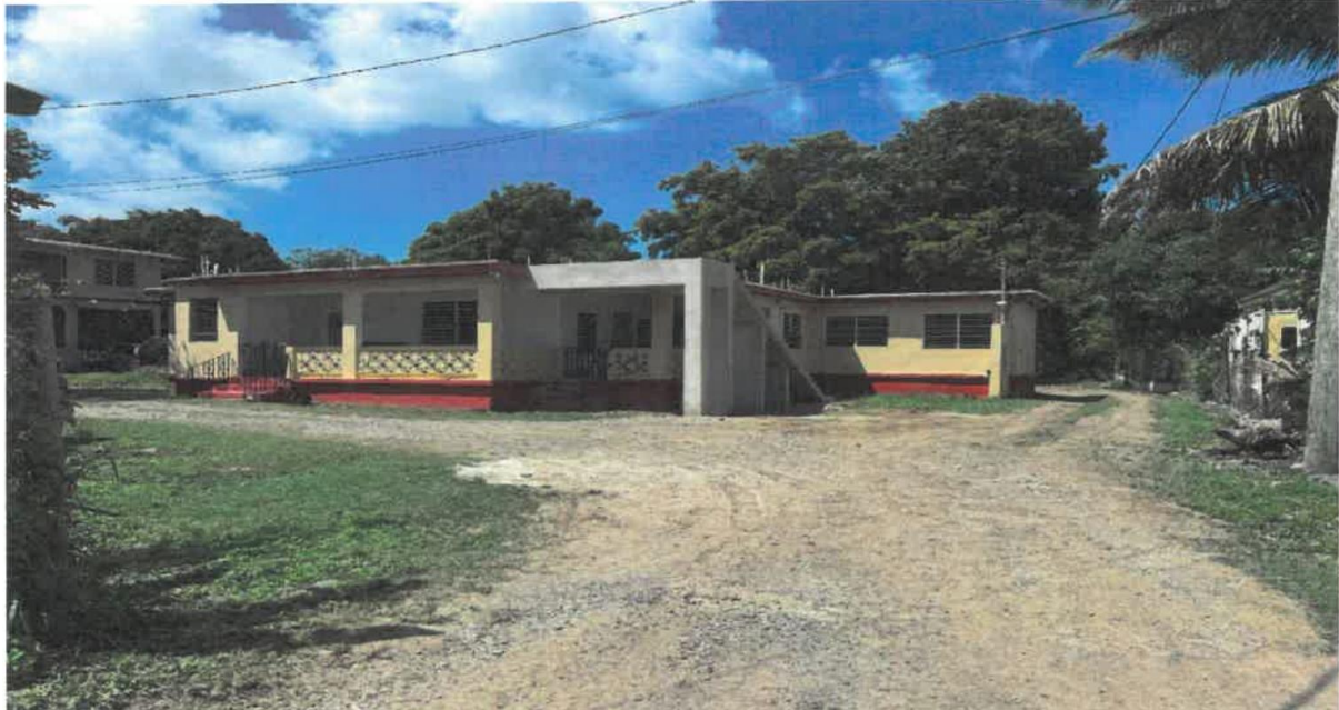
Site photo- Occupied residential building
