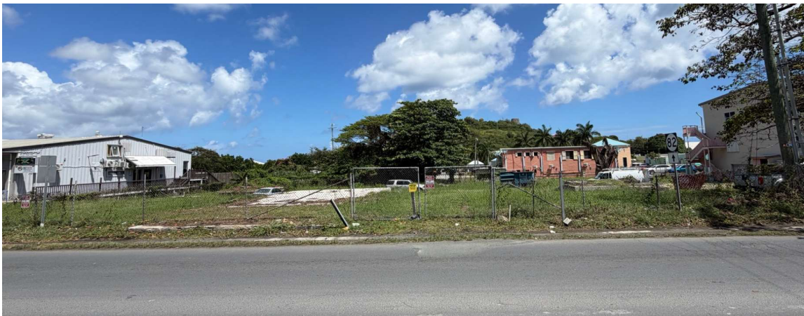
Site photo-undeveloped lot
