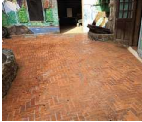
After — Restored brickwork
