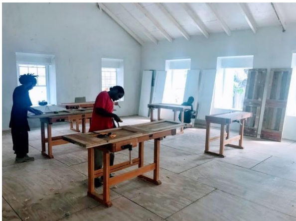
IH Apprentices constructing shutters
