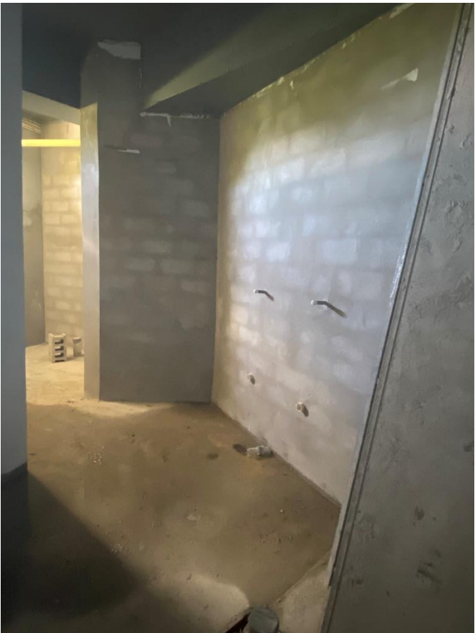
Shower Area in Locker Room
