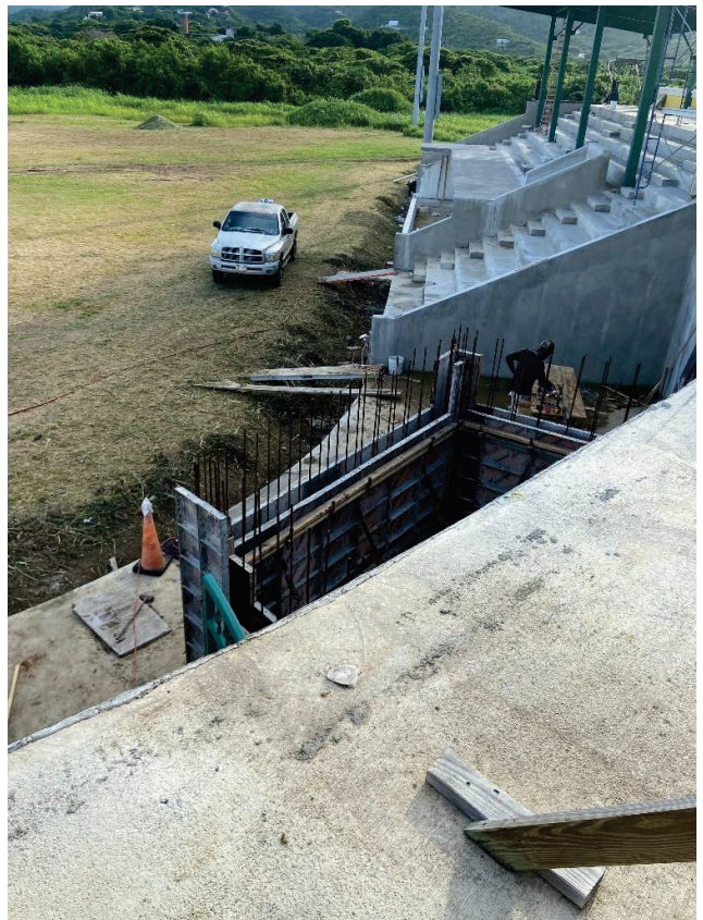
Press Box and A/V Booth – Formwork
