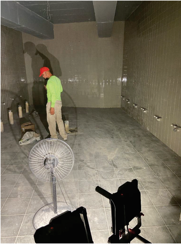
Male and Female Restrooms – Floor and Wall Tile Installation Field Level
