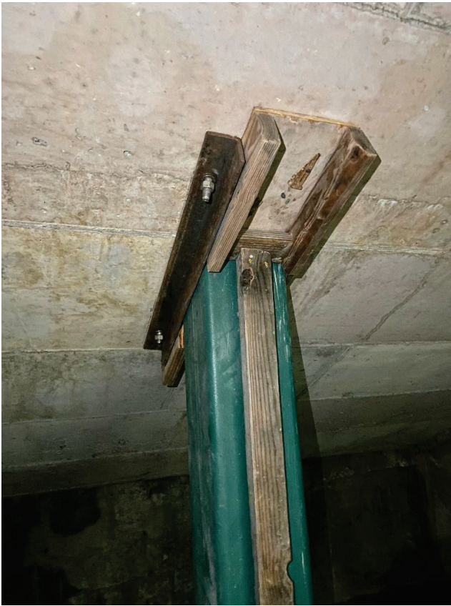
Bleacher Roof Column – Formwork to Fill Slab Penetration
