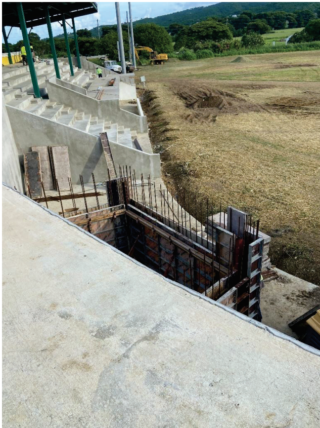
Press Box and A/V Booth – Formwork
