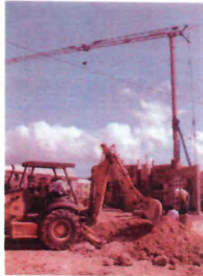
Site electrical install at Louis E. Brown, Est. Paradise, St. Croix
