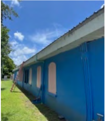
Rivera Roof and Gutter Replacement
