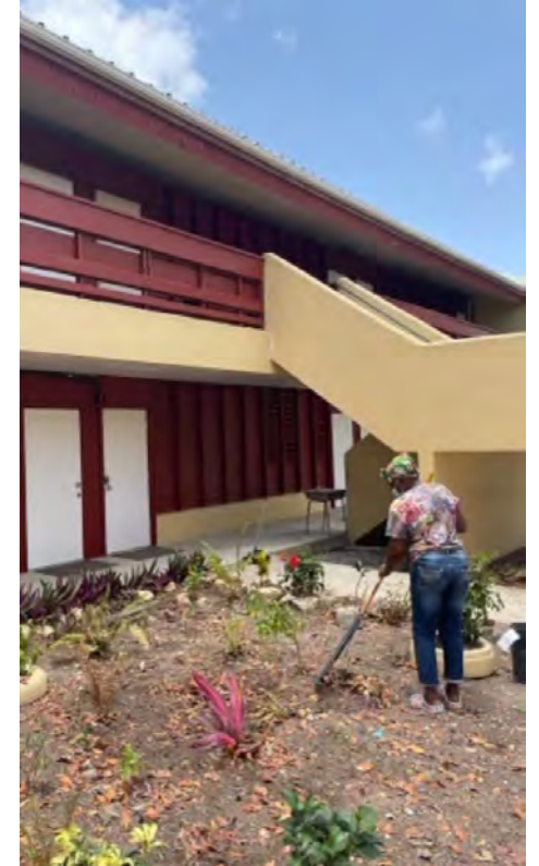
Lew Muckle Painting and AC Install
