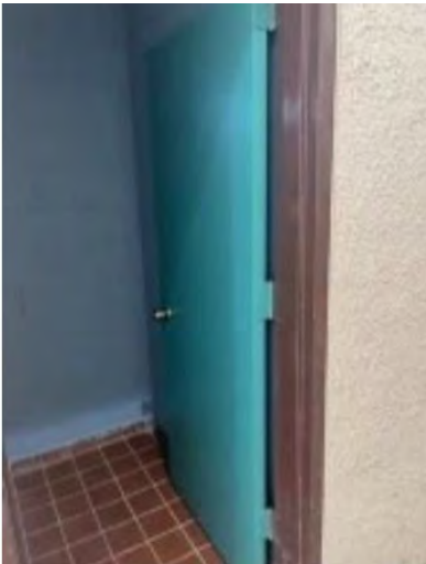
John Woodson Bathroom and Stage Repair
