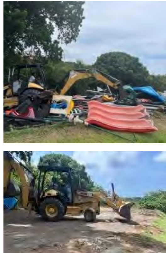
Pearl B Larsen Playground Demolition
