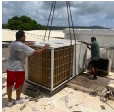
Alfredo Kitchen HVAC Replacement
