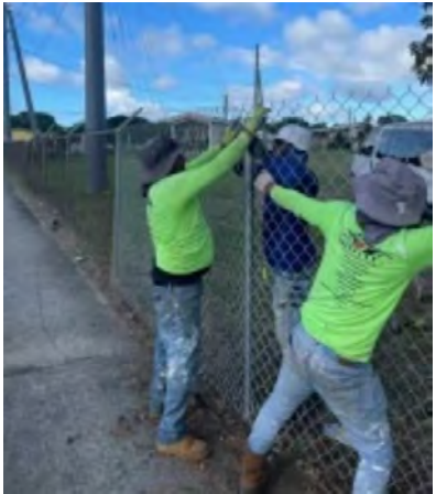
Woodson Fence Replacement
