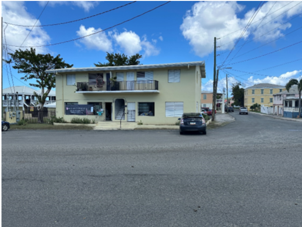
VIEW LOOKING NORTH AT THE CORNER OF FISHER STREET & STRAND STREET
