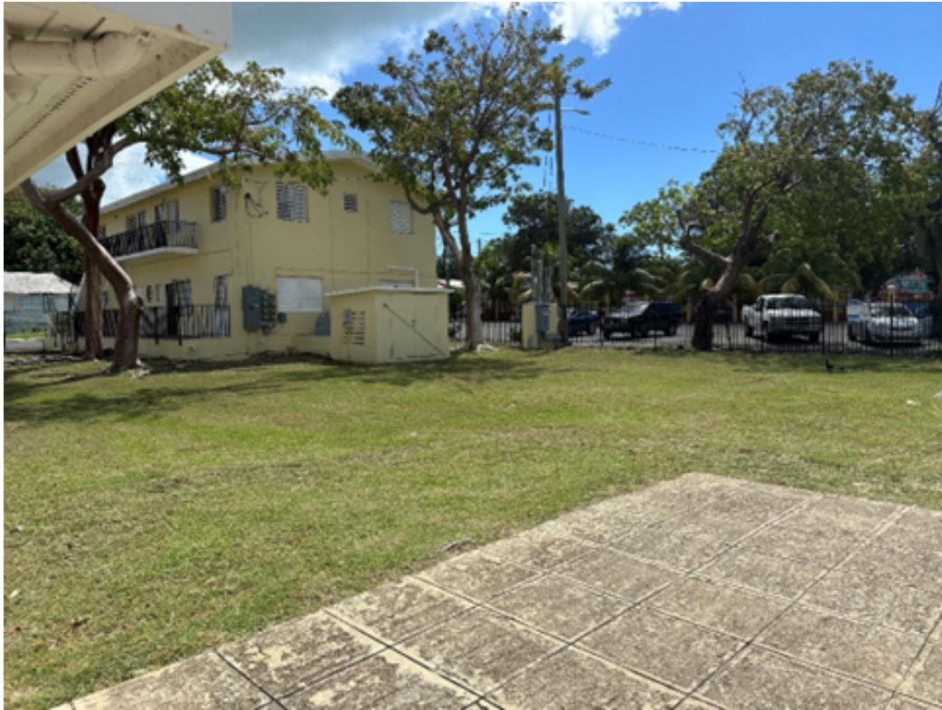
VIEW LOOKING EAST FROM 37 STRAND STREET
