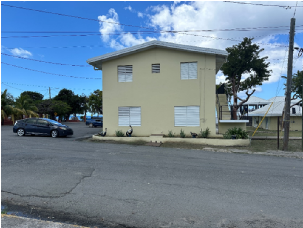
VIEW LOOKING WEST FROM STRAND STREET
