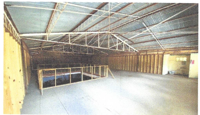
Inside Bldg. #20 – 2 nd Floor Facing Away from Prince St.
