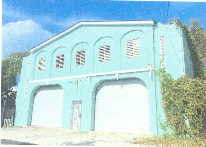
Front of Bldg. #20
