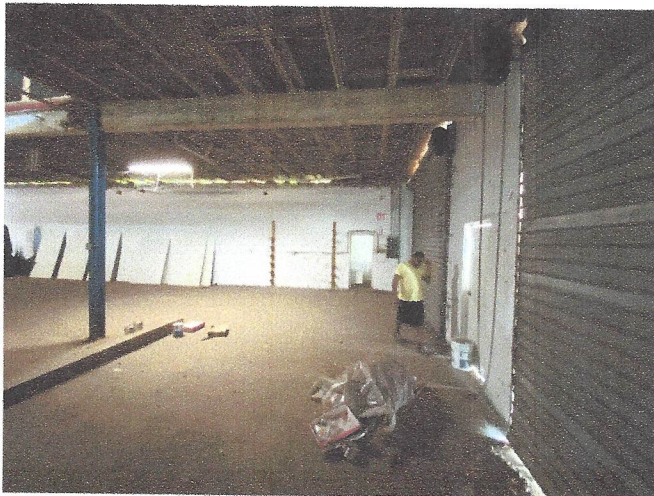
Inside Building #20 – Facing Away from Office
