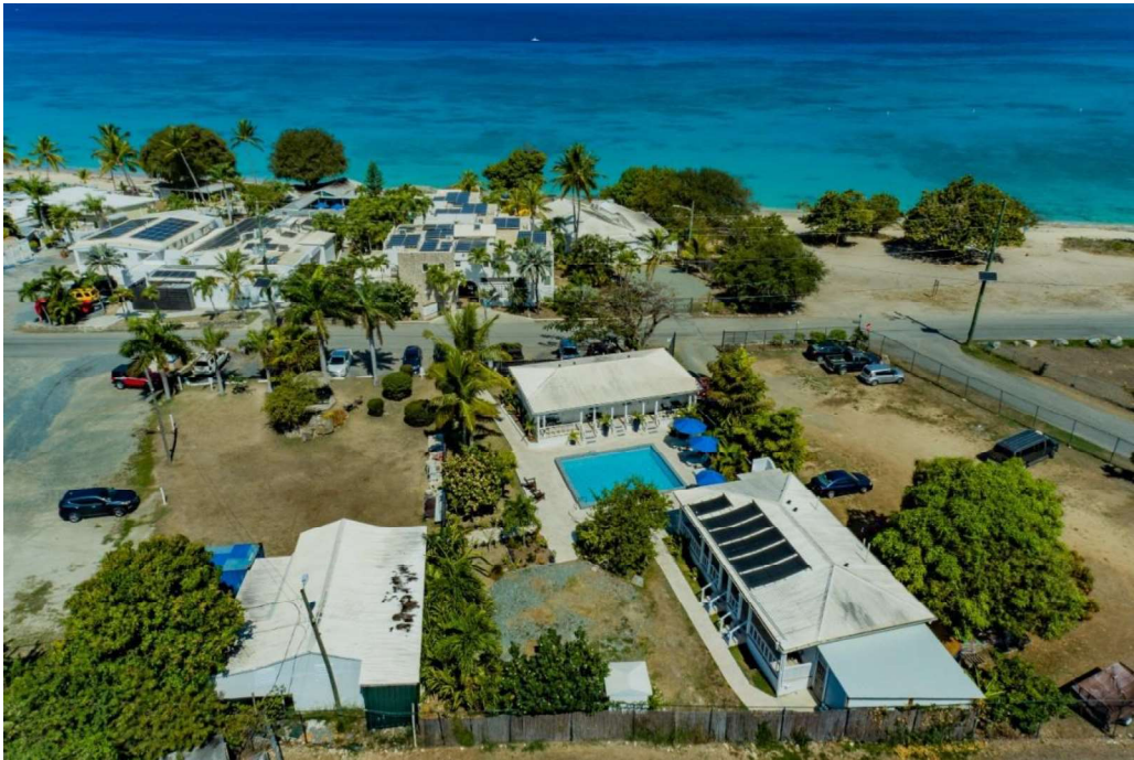
Photo of current site condition
