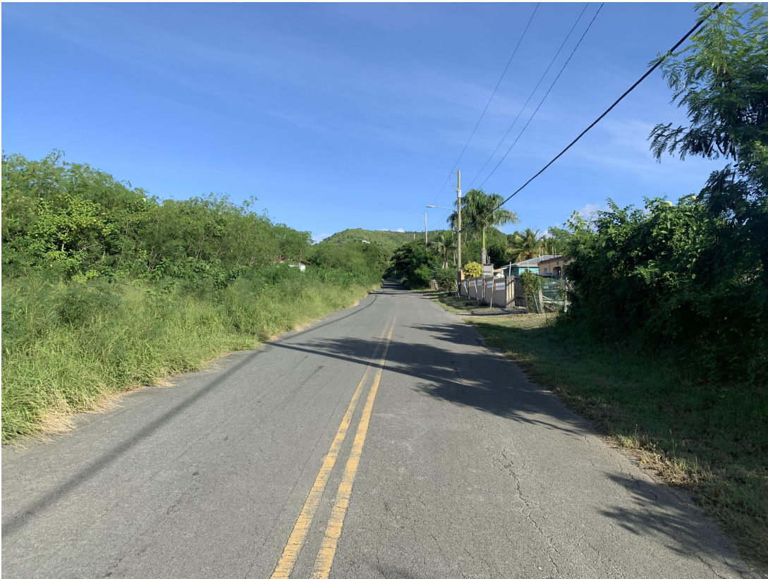
VIEW ALONG MOUNTAIN ROAD LOOKING NORTH
