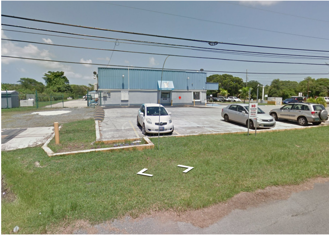
VIEW ALONG MOUNTAIN ROAD LOOKING EAST
