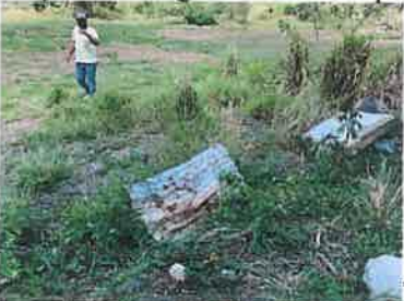
There are piles of rubble on the edge of the property which may have originated on the property.
