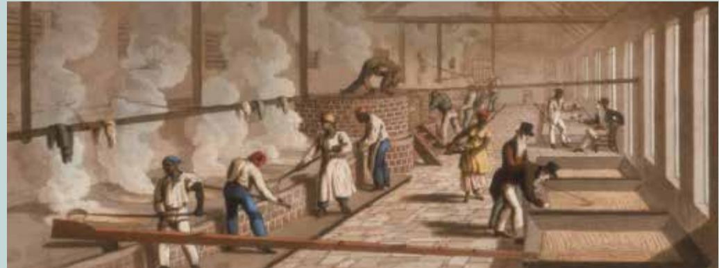
A period drawing showing the process of boiling, skimming, and cooling of sugar in a factory (St. Croix Landmarks Society).
