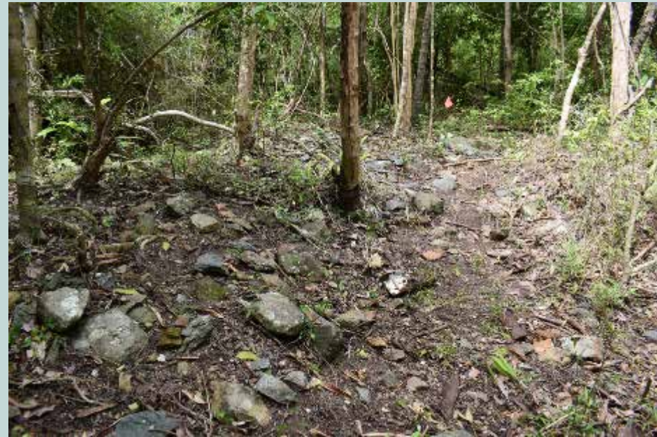
Stone foundation remnants in the enslaved laborers' village (Quinn Evans 2021).
