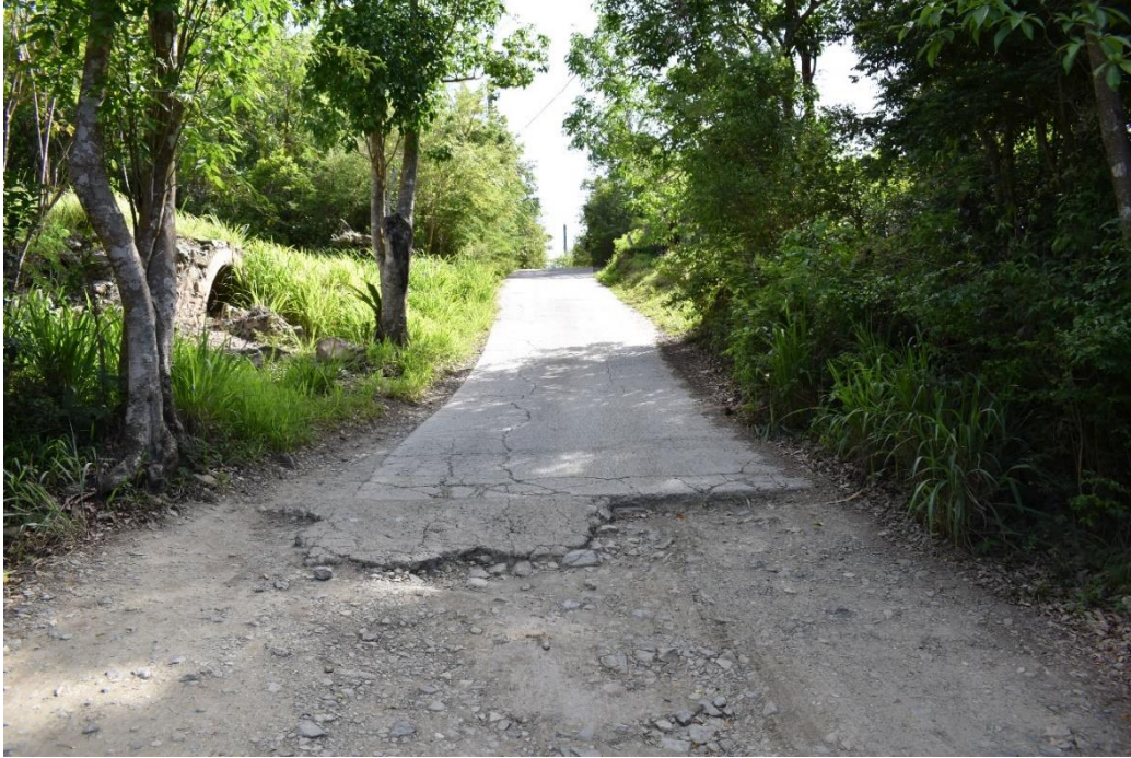
Slope up to the animal mill and windmill along John Head Road, looking north (Source: Quinn Evans)
