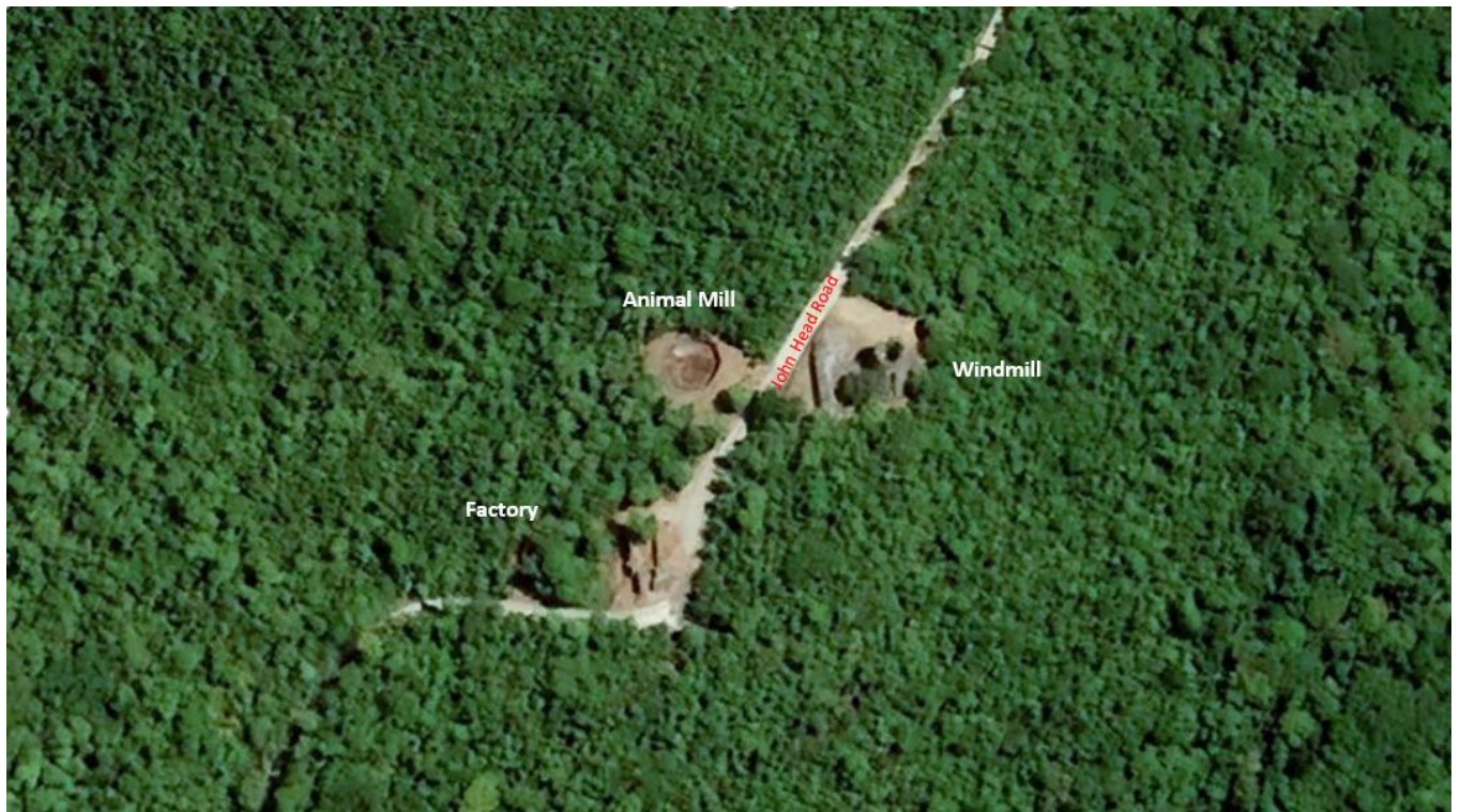
Aerial view of the spatial organization of Estate Catherineberg (Source: Google Earth)
