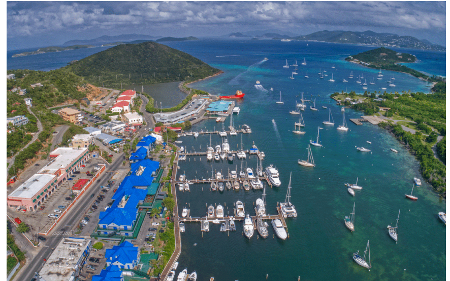
High volume traffic area with mixed uses in Red Hook, St. Thomas (source: stthomassource.com)
