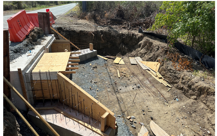
Top: Construction practices in sensitive areas
