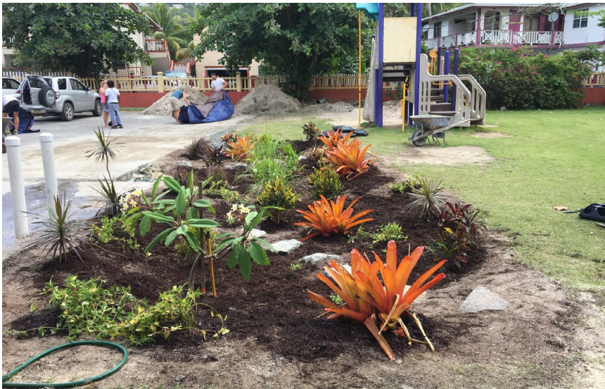
Top: Landscape design capturing runoff from driveway Bottom: Raingarden captures stormwater runoff
