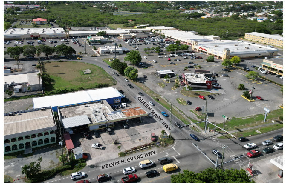
Above: Existing conditions, Sunny Isle Shopping Center
