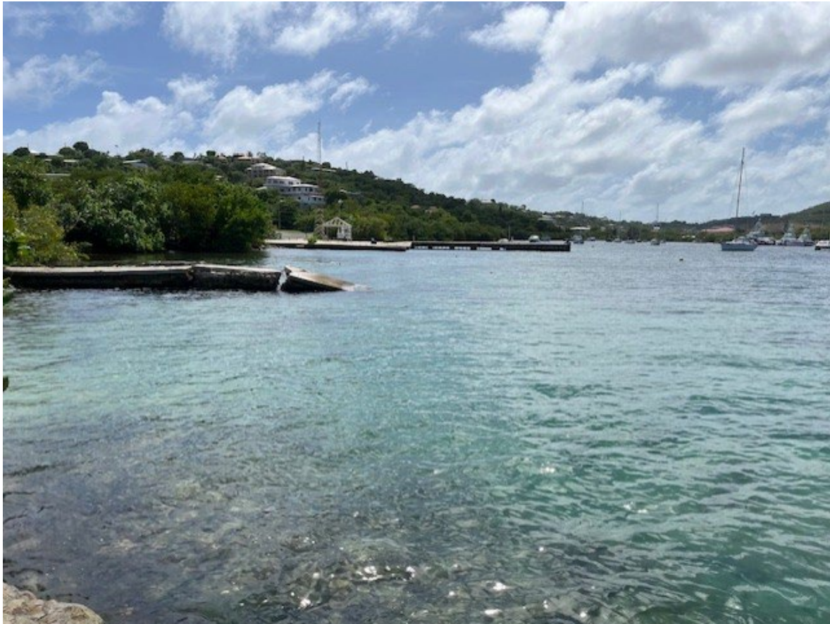
LOOKING WEST INTO VESSUP BAY
