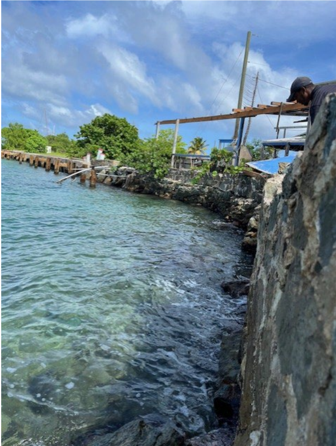
MARINA BULKHEAD AREA
