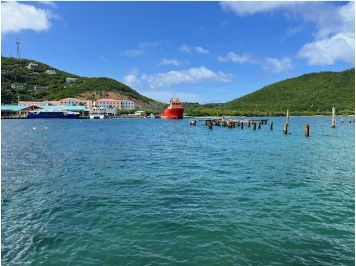
LOOKING NORTH AT REDHOOK FERRY TERMINAL
