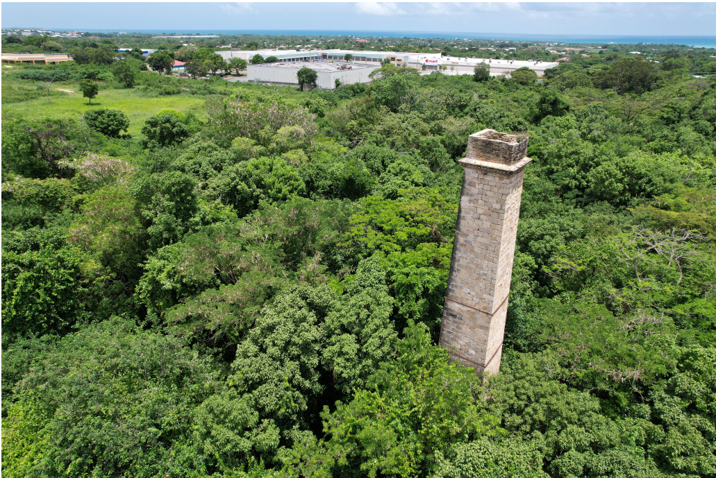
AERIAL VIEW LOOKING SOUTH-EAST
