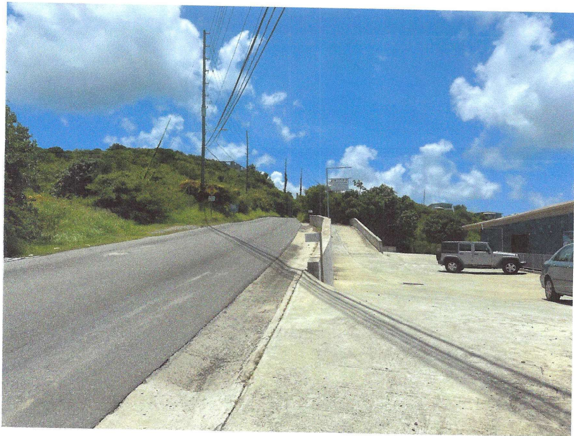
Parcel No. 41-5-1 Estate Frydenhoj, St. Thomas – East View
