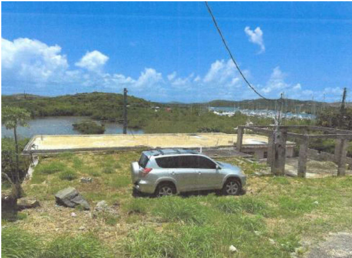
Photo of current site condition- abandoned residence
