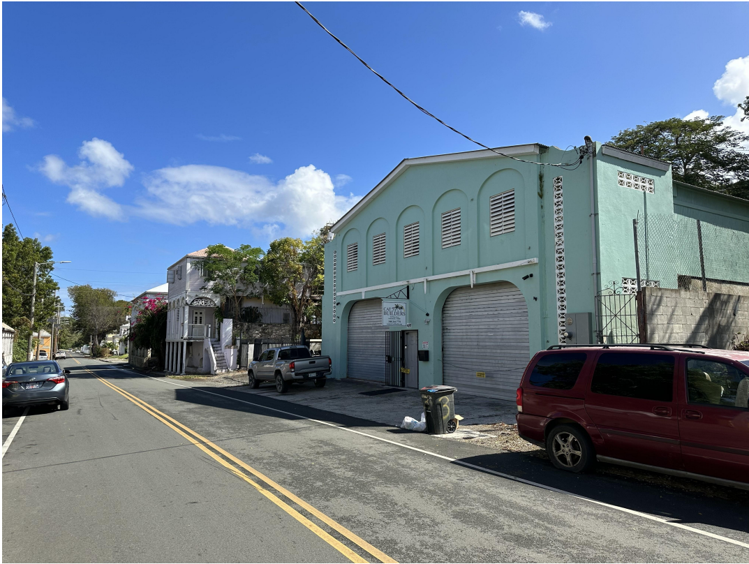
VIEW LOOKING NORTH FROM HOSPITAL STREET
