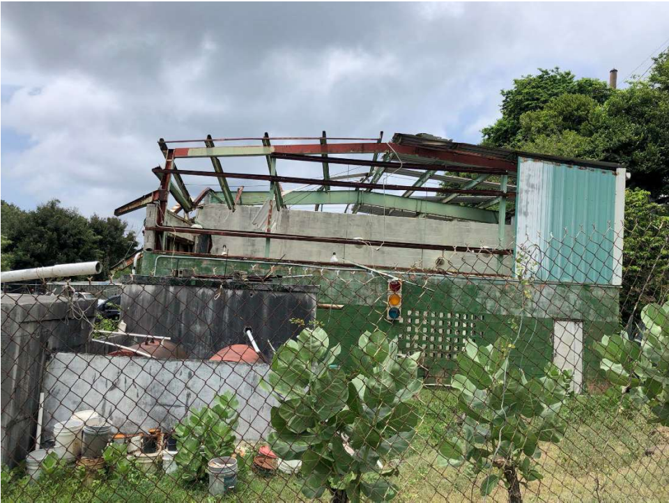
Figure 12: View From Public Road
