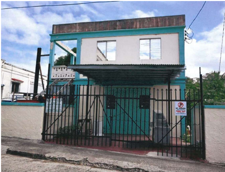
Photo of current site condition
