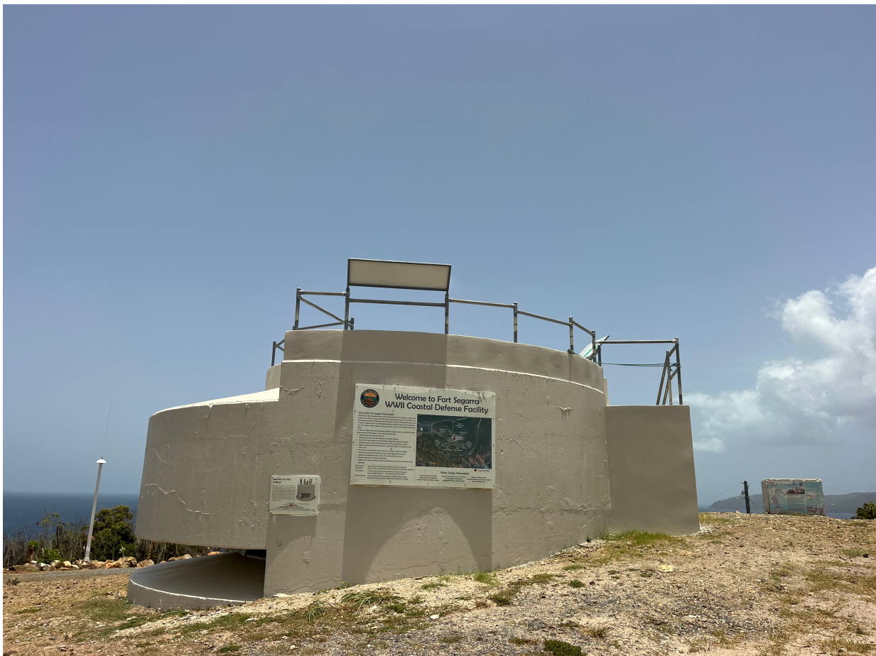
Fort Segarra after extensive rehabilitation through a DPNR sub award grant
