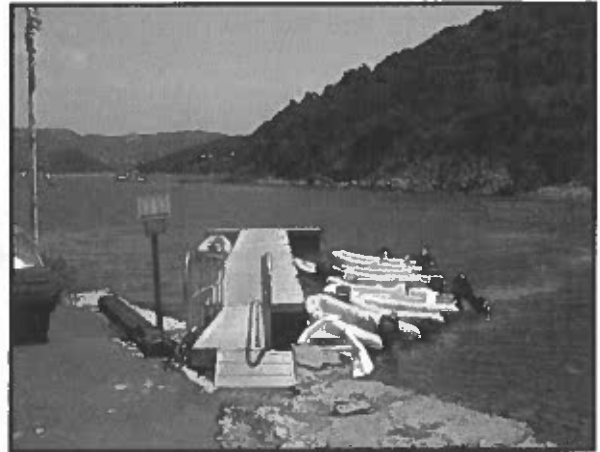
Figure 2-3 Temporary dock at the Water Island passenger ferry dock area
