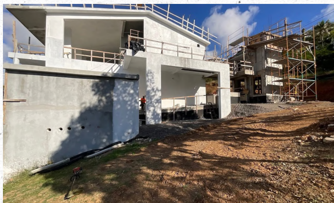
Dilsa Capdeville Head Start Facility (STT): 90% Complete ($11.0M)
