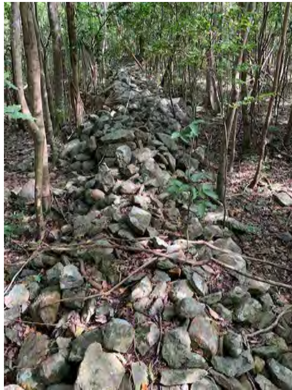
Stone Wall Surrounding Old Farm Area on Southeast Part of Subject Tract
