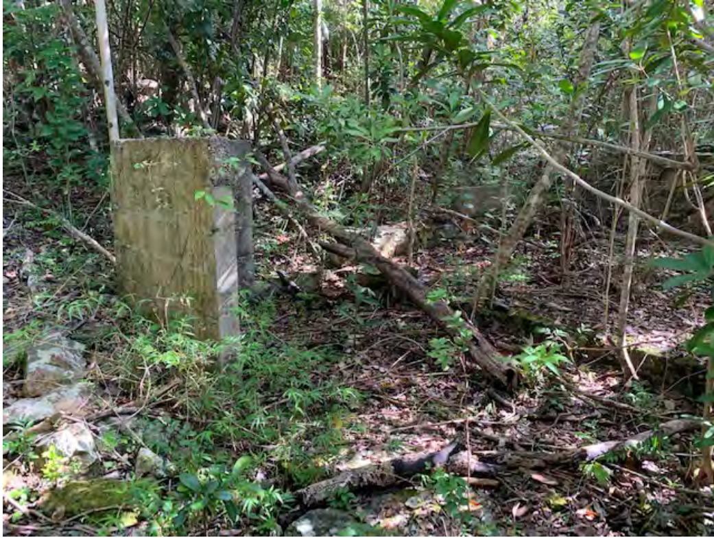
Concrete Block Wall & Foundation on Southeast Part of Tract 01-137A
