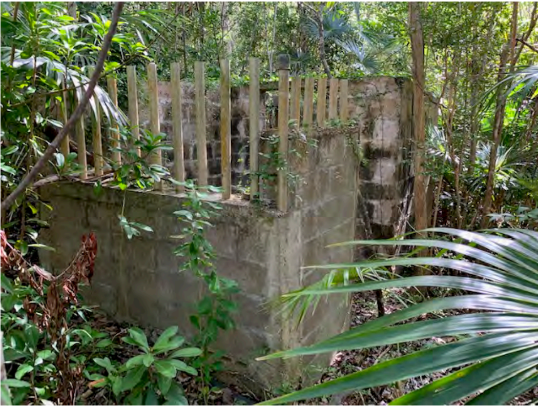
Roofless Cinder Block Structure on Southeast Part of Tract 01-137A
